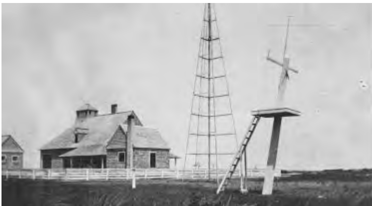
FIGURE 22. Looking east toward the Portsmouth Life-Saving Station and kitchen, including the station's wreck pole, coastal warning display tower, and oil house, circa 1916. Wood board fencing enclosed the complex.
