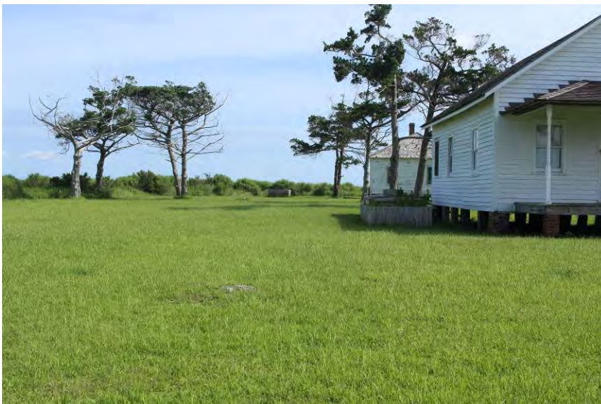
FIGURE 138. An above-ground septic tank and wooden enclosure at the Carl Dixon House.
