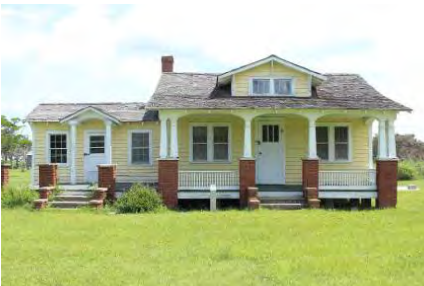
FIGURE 47. The same view of the Harry and Lida Dixon House as Figure 46 . Note the loss of the decorative trellis on the porch, the pickets along the side addition, the low fencing in front of the house, and the change in mortar associated with the brick.
