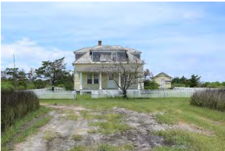
FIGURE 54. The Styron and Bragg House. The second story has been shingled, and the lattice under the porch has been altered, a picket fence has been added, and there has been some loss of vegetation since previous documentation.
