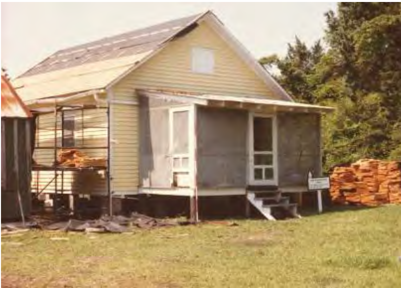
FIGURE 73. The north facade of the Carl Dixon House, circa 1979.
