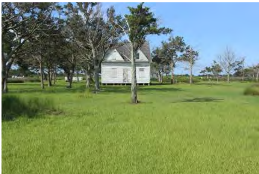
FIGURE 63. The Walker and Sarah Styron House, illustrating changes in vegetation, and the loss of the long building extension (kitchen wing) to the right of the Walker and Sarah Styron House. Note the replacement of the central dormer with two dormers and alteration of the porch posts and railing. Woodwork beneath the porch is no longer present.
