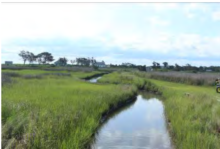
FIGURE 107. Drainage channel along the northern portion of Haulover Point Road by the WPA for mosquito control.
