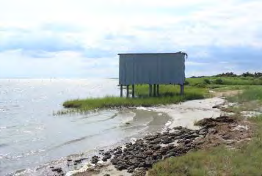
FIGURE 78. The Frank Gaskill shed on raised wood piers on the inlet shore.
