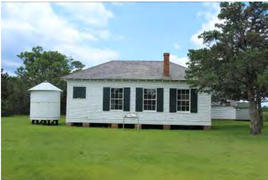
FIGURE 152. The original entrance to the Schoolhouse was at the end wall where the cistern is now located. This former entrance was closed up when the building was converted to living quarters circa 1940s.
