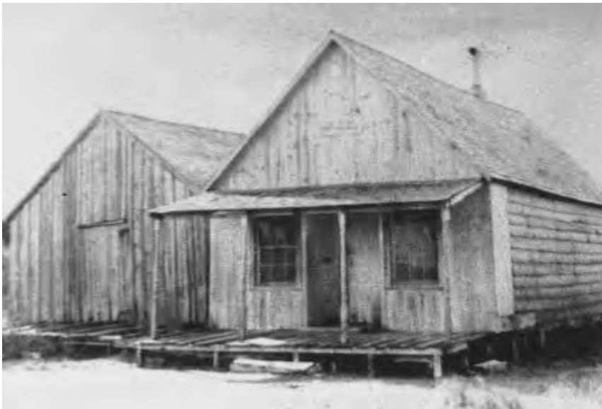
FIGURE 50. Post Office and General Store with addition, circa 1930s.
