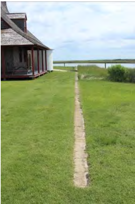
FIGURE 113. View northeast along the seawall and ramp that afforded access to Coast Guard Creek for Life-Saving Station needs.
