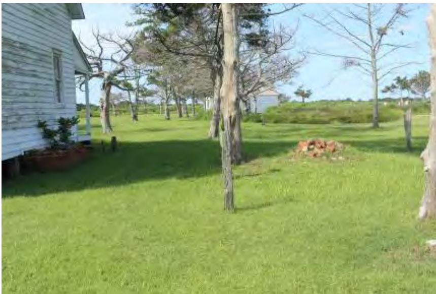
FIGURE 65. Looking across the north façade of the Walker and Sarah Styron House, illustrating changes in the building roof line, the loss of a step leading out of the building, and the dramatic loss of vegetation behind the house. There are several wood posts and a pile of bricks that indicate the outline of the former kitchen addition.
