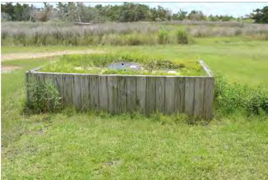
FIGURE 114. Above-ground septic systems, such as this one associated with the T.T. Potter House, are typically used for wastewater treatment and management in association with most buildings in the district.
