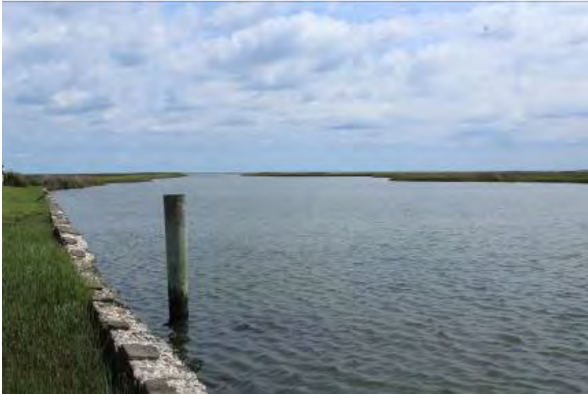
FIGURE 32. View along the concrete seawall and wooden mooring posts in Coast Guard Creek at the Portsmouth Life-Saving Station.
