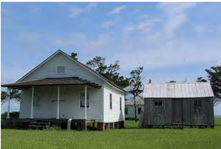
FIGURE 75. Carl Dixon House and summer kitchen. Changes since 1979 include loss of the front porch, replacement of the roof, and a change in paint color. Changes to the summer kitchen includes the boarded window, different cladding of the shed, the addition of a vent pipe, replacement of the door, addition of wooden steps, and lack of paint.
