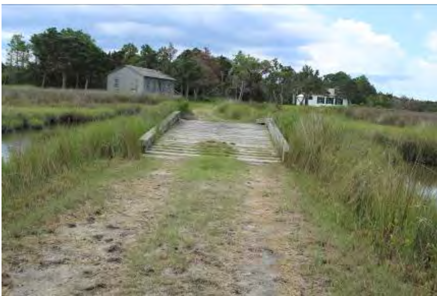
FIGURE 102. Access road and bridge to the Cecil and Leona Gilgo House and the Portsmouth Schoolhouse.
