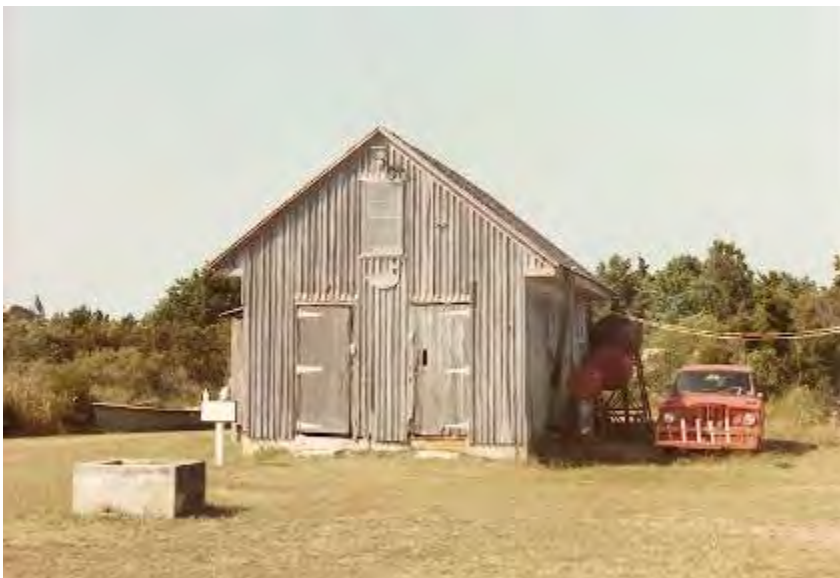
FIGURE 30. The Portsmouth Life-Saving Station stable, circa 1983.
