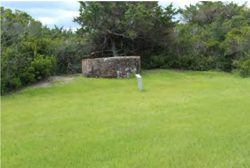
FIGURE 140. Cisterns like the U.S. Marine Hospital structure shown here were used to store rainwater on the island and are the primary source of fresh water.
