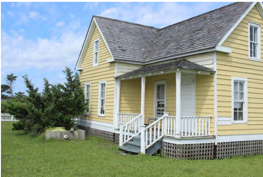
FIGURE 137. An above-ground septic tank and wooden enclosure at the Henry Pigott House.
