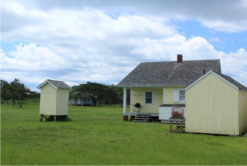
FIGURE 142. The Jesse and Lillian Babb water box is visible attached to the back of the house, to the right of the rear porch stairs.
