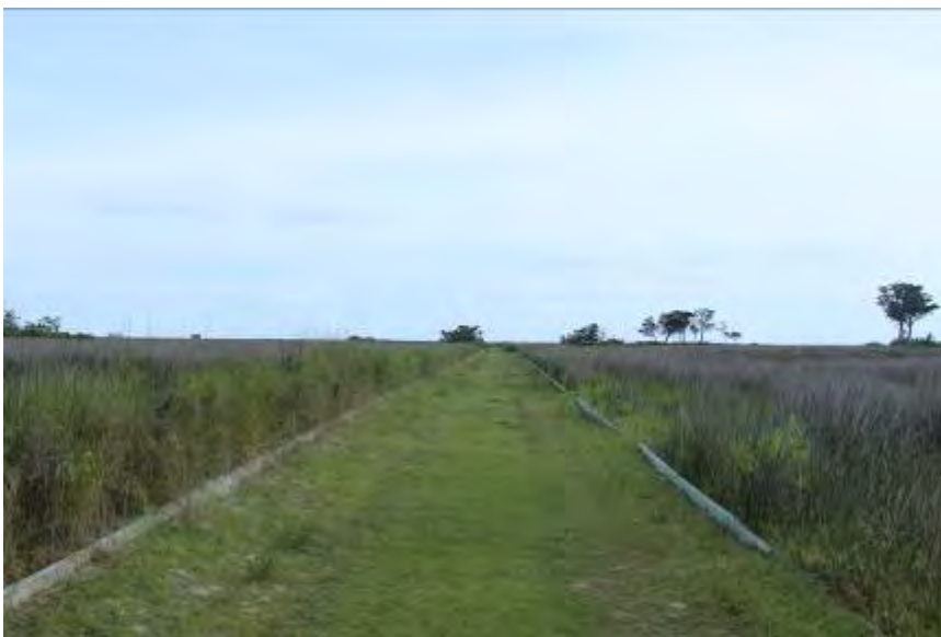
FIGURE 149. Sections of Haulover Point Road are wood lined on both sides.
