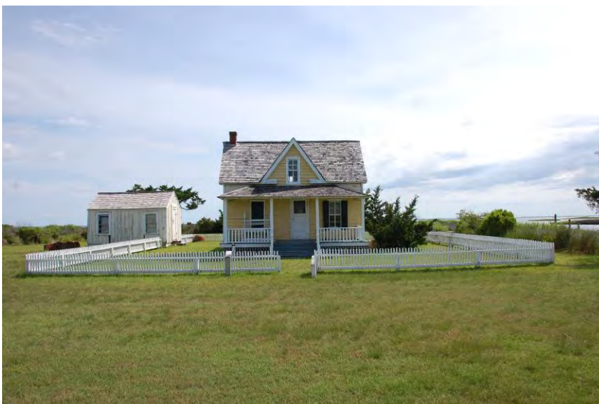
FIGURE 151. Most of the properties located within the historic district, such as the Henry Pigott House shown here, are maintained through close mowing of the grass to establish an open precinct around the buildings.
