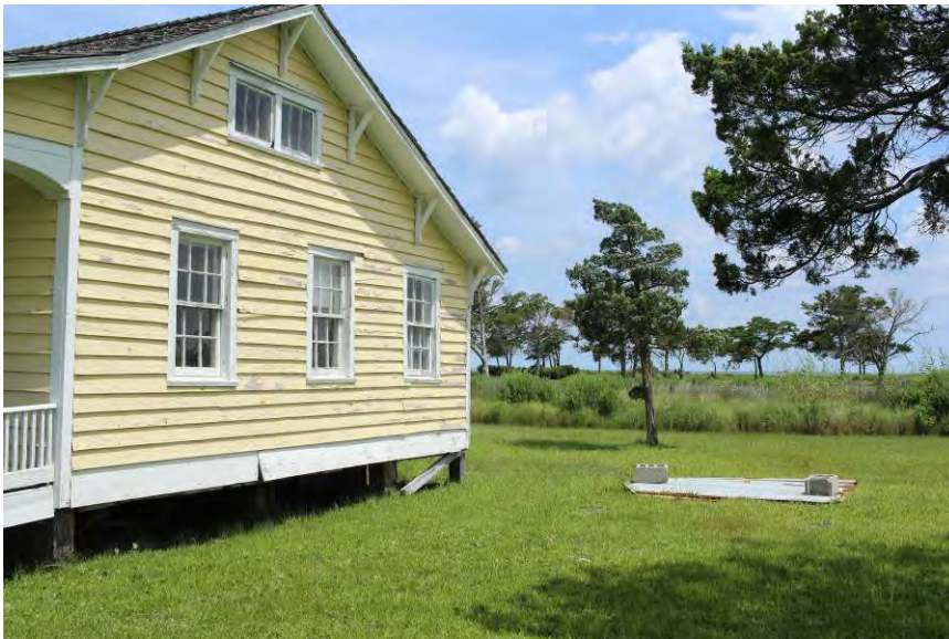
FIGURE 136. The Harry and Lida Dixon House metal septic cover on right.
