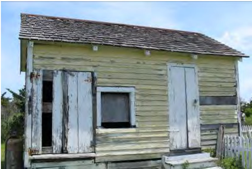
FIGURE 58. The Styron and Bragg shed.
