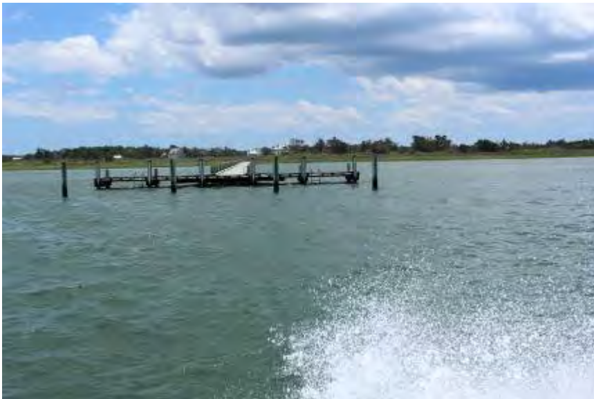
FIGURE 88. The T-shaped dock and boardwalk at Haulover Point.
