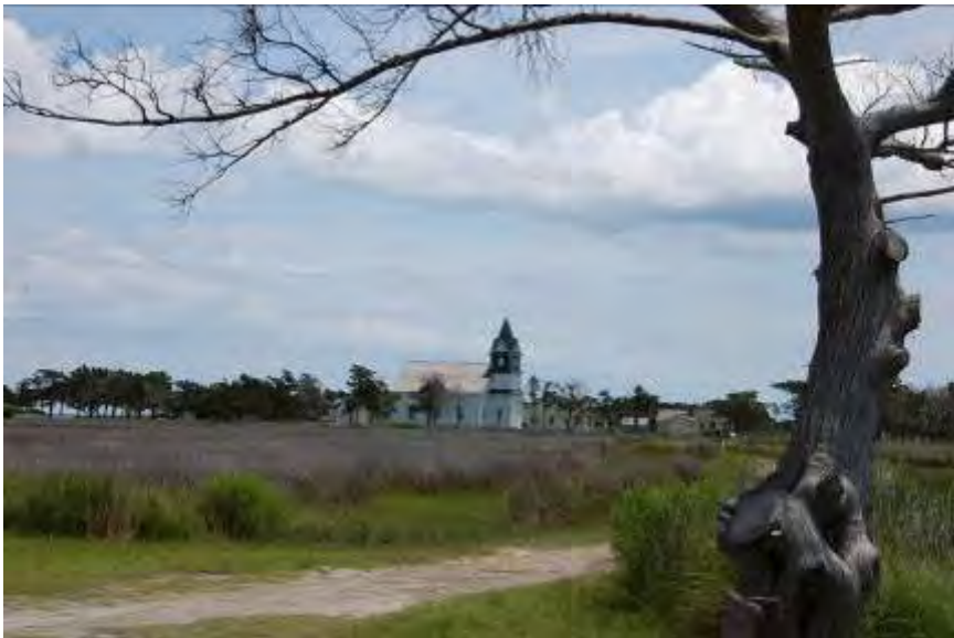
FIGURE 160. View towards the Portsmouth Methodist Church.
