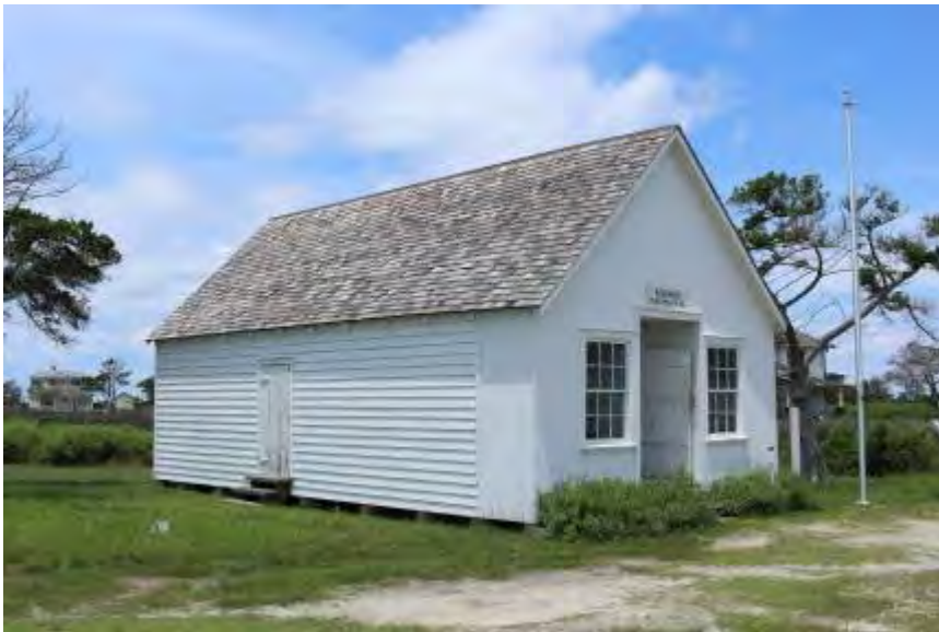
FIGURE 52. The Post Office and General Store, showing changes since the 1930s including the loss of the addition and removal of the porch and overhang. The vent pipe in the rear is also gone.
