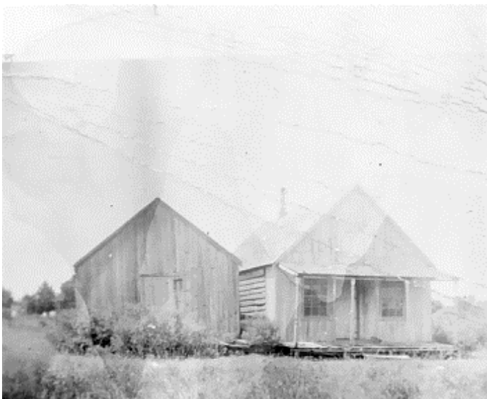
FIGURE 51. View west toward the Post Office and General Store, date unknown.
