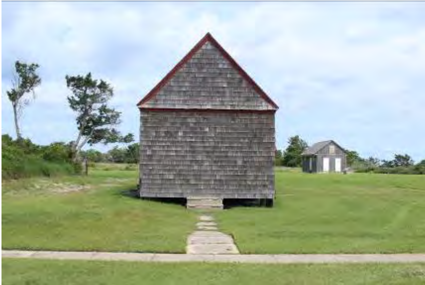
FIGURE 105. Concrete walks extend between the Portsmouth Life-Saving Station and summer kitchen, as well as into the landscape.
