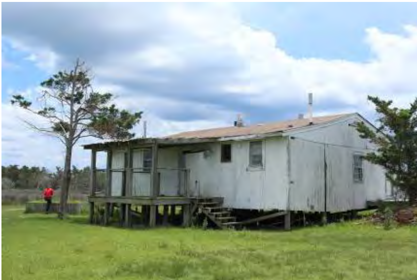
FIGURE 80. The T.T. Potter House. There is an addition to the building along its rear facade, the screen porch has been removed, and the siding has been replaced.
