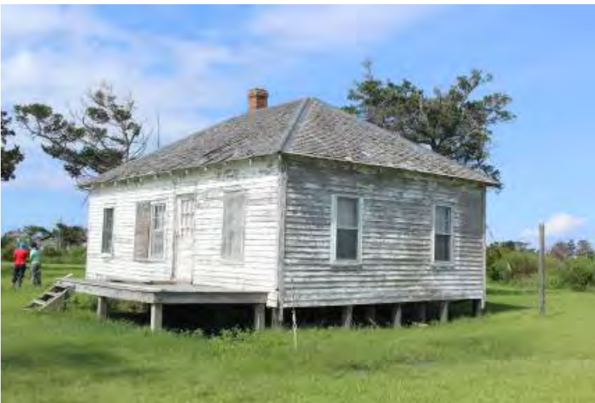
FIGURE 77. The Frank Gaskill House, illustrating the loss of the roof overhang associated with the porch, and the wood stair and landing along the side/rear of the house. The vegetation is now mown cool-season grass, whereas the earlier view suggests native warm-season grasses were present previously. Cabling is currently stabilizing the structure.
