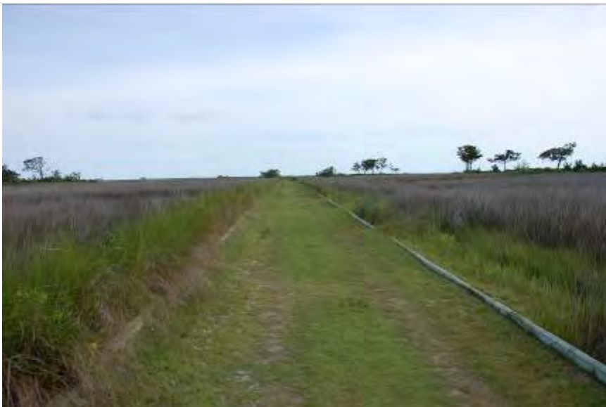
FIGURE 92. View north along Haulover Point Road.
