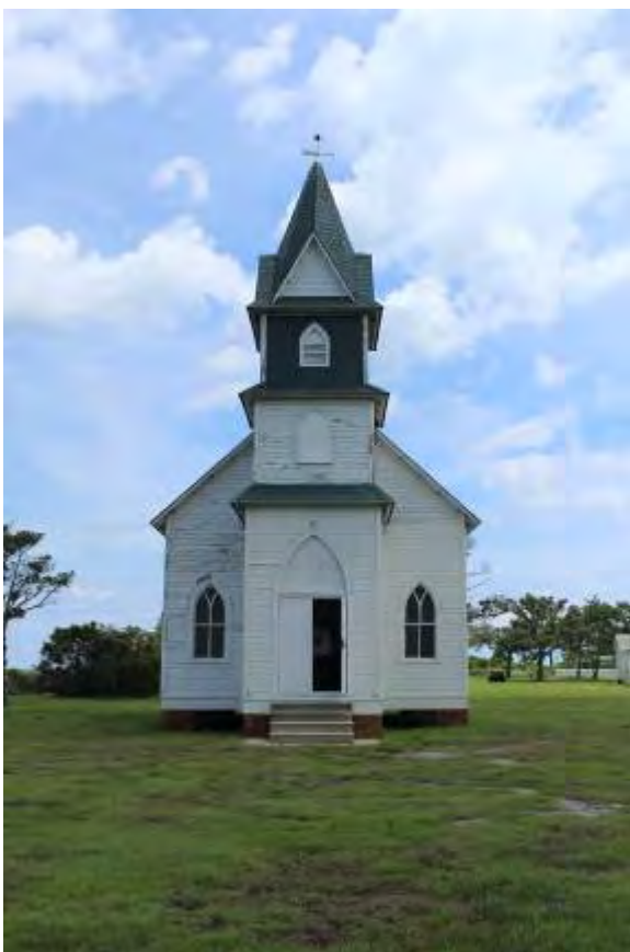
FIGURE 39. The front façade of the Portsmouth Methodist Church.
